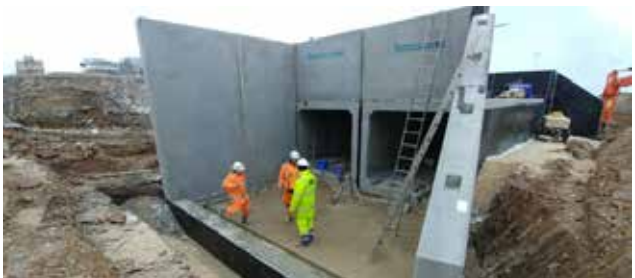
Box culvert with wing walls
